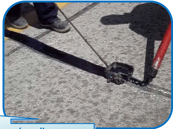
Routing, clearing and crack sealing
