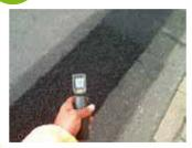
An Infrared Thermometer is used to check the temperature of the repair area, material temperature should be between 70-100°C to provide the best compaction conditions.
