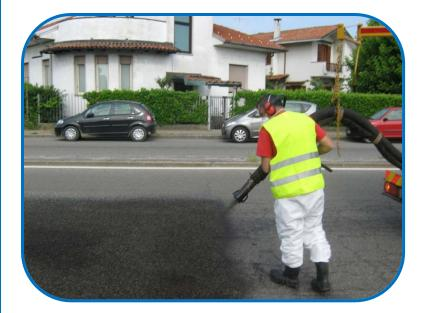
Laying of grit mixed with modified bitumen emulsion
